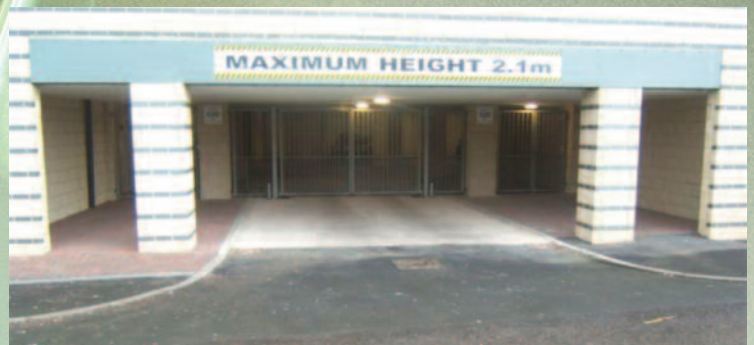
Security swing gates for underground carpark.
