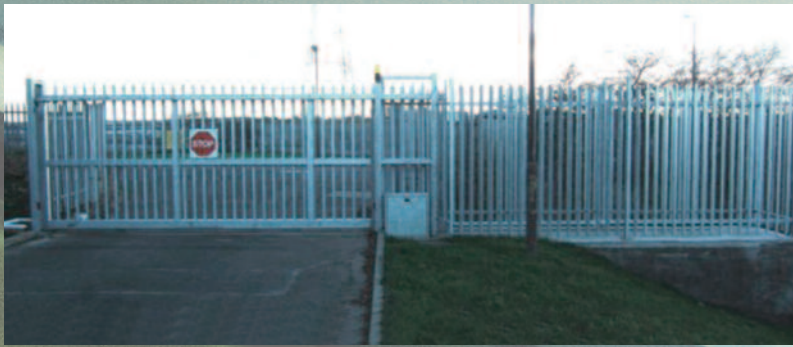
Security sliding gate for Northumbrian Water.
