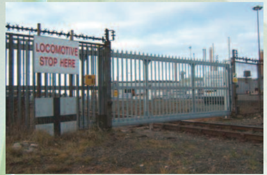
Security sliding gate for Rio Tinto across railway line.
